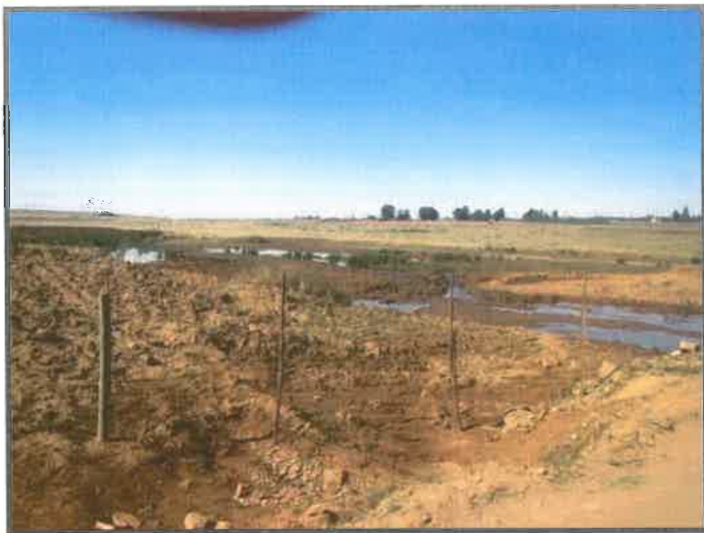
Photograph 9.1-16: The road works have created an unpleasant sight in the impeding of the wetland with the disposal of soil and rubble on the edges of the as wetland (north west side).
