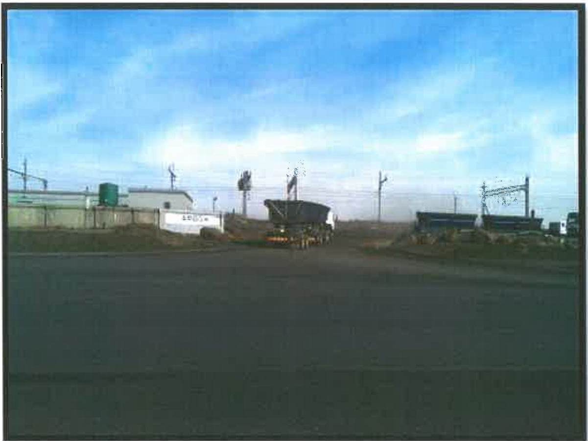
Photograph 3.1-1: View of Site Activities
