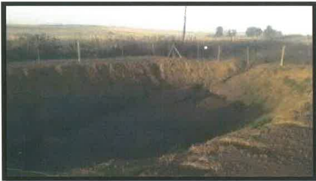
Photograph 5.1.3-1: Pollution Control Dam on site.
