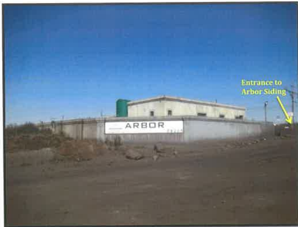
Photograph 9.1-18: The entrance to the Arbor Siding on the R555 road towards Delmas.
