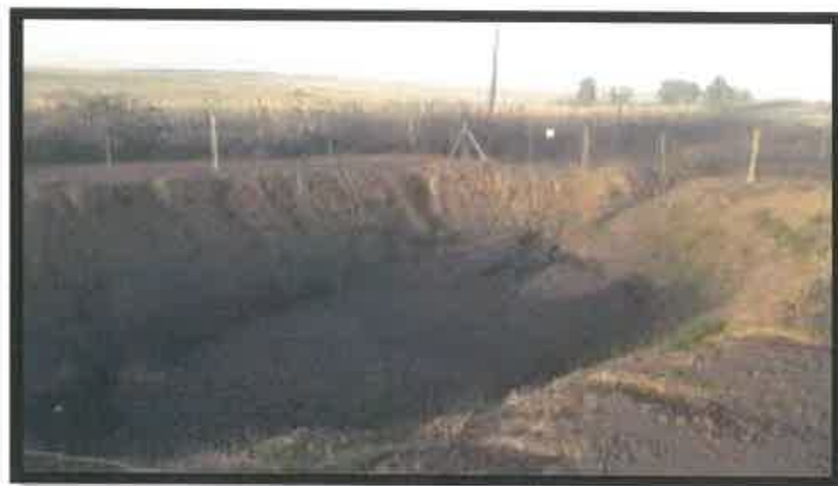
Photograph 5.1.3-1: Pollution Control Dam on site.
