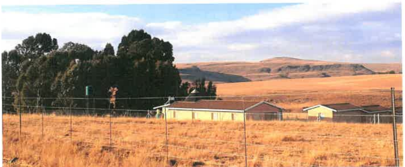
Typical example of structures to be built as part of relocation programme.
