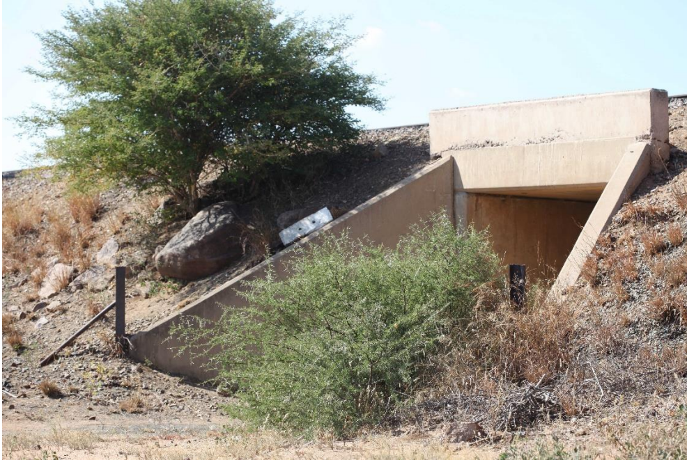
Photo 10 Streamcrossing No 1 at the site in winter. Photo: R.F. Terblanche
