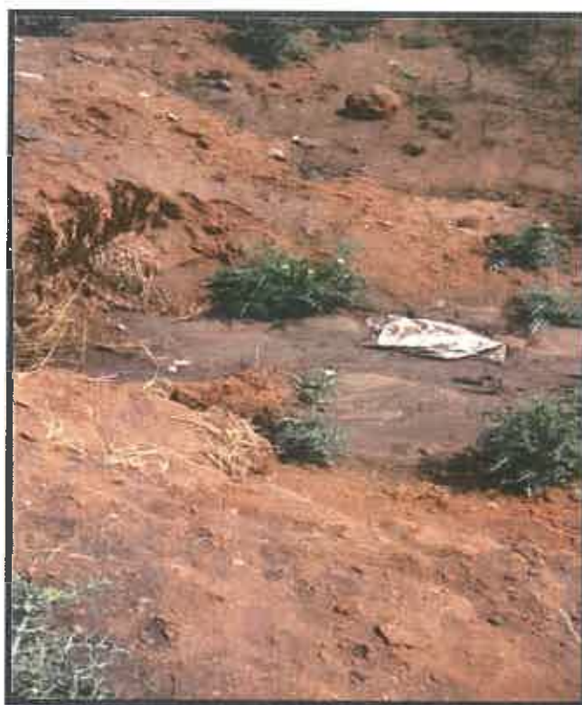
Figure 13: Stormwater colbet from R555 used to drain stormwater from the operational site.
