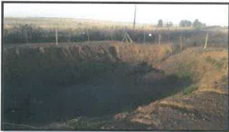
Figure 10: Slurry Control dam within Arbor siding (Image ©MYEZO).
