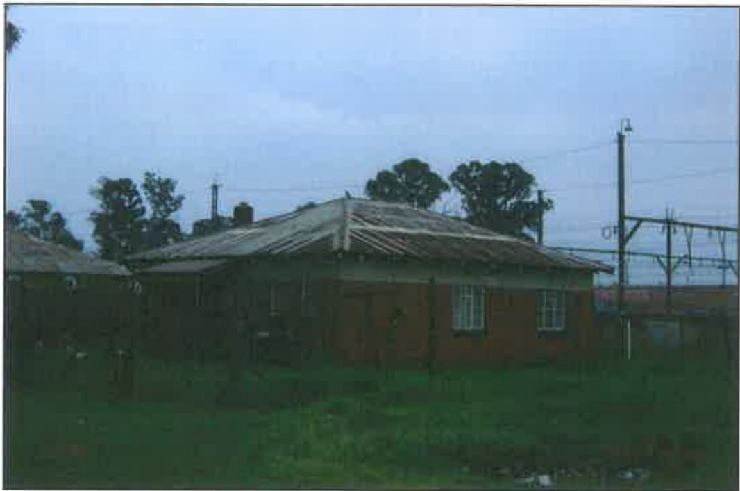
Figure 12. Typical station house at Delmas
