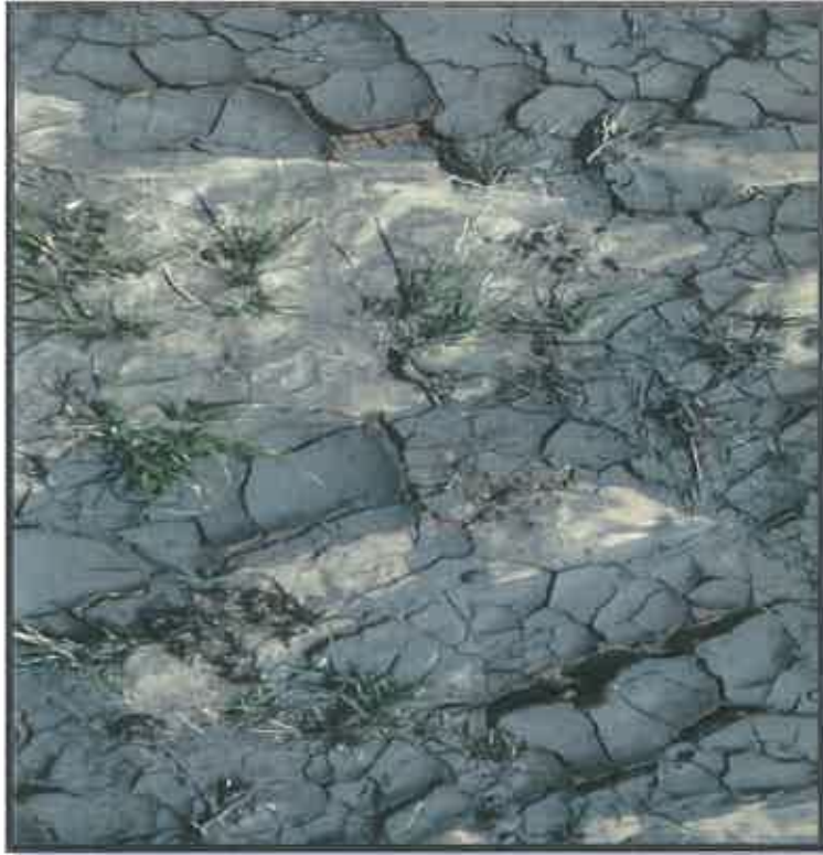
Figure 16: Dried coal dust residue stormwater.
