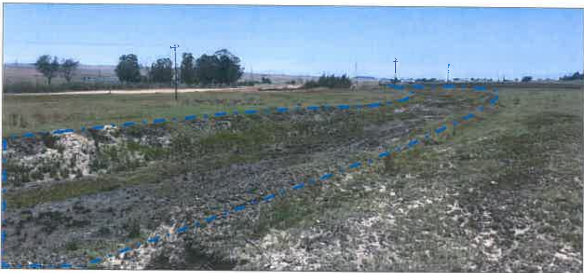
Figure 16: Old railway siding on the eastern periphery that is not in use anymore acts as an effective, large drainage canal. Note that the whole of the old siding is located within the seepage wetland
