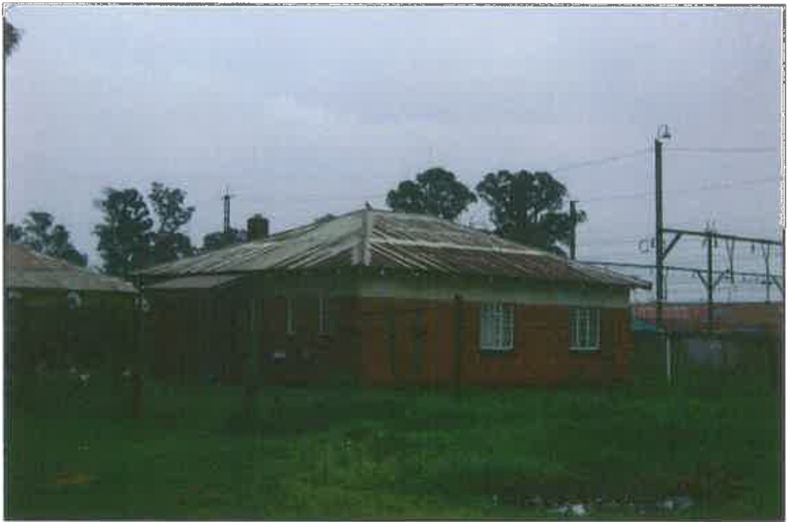
Figure 12. Typical station house at Delmas
