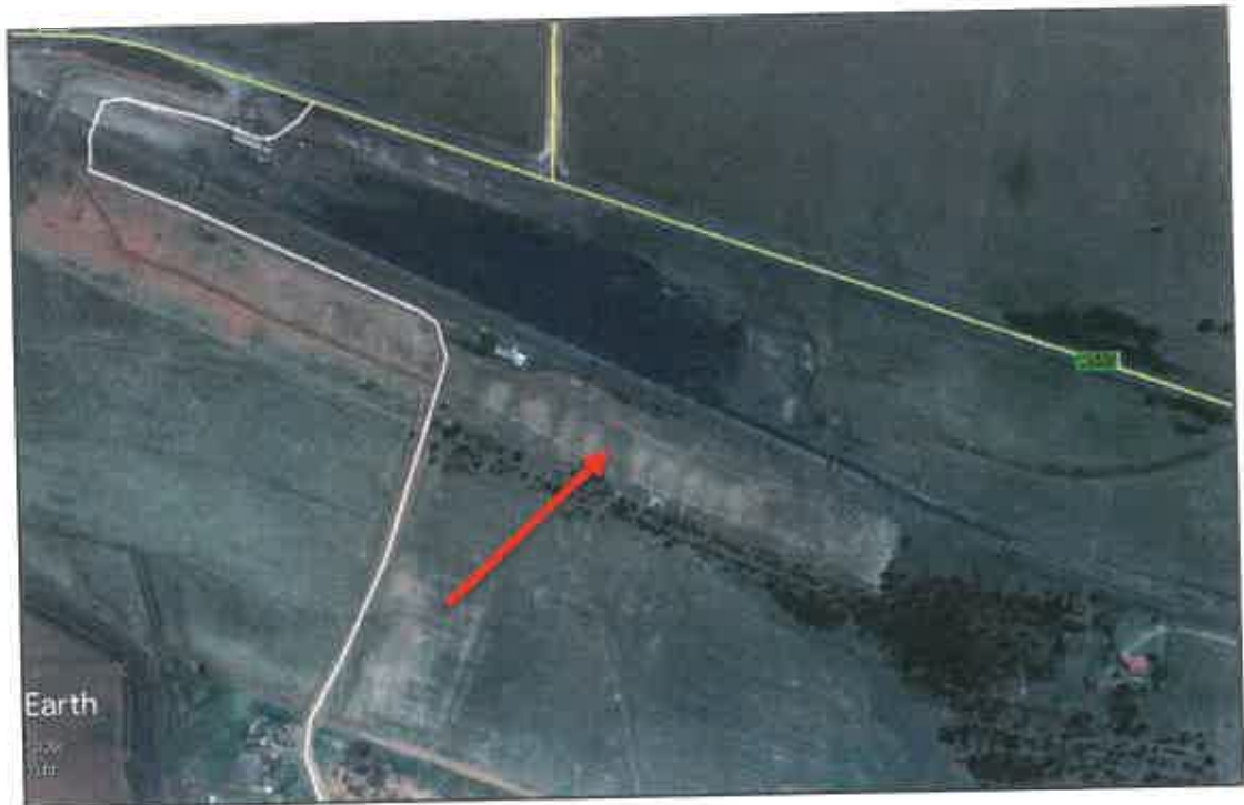
Figure 14. Indicating that the station houses has been demolished (2018) (Image: Google Earth)
