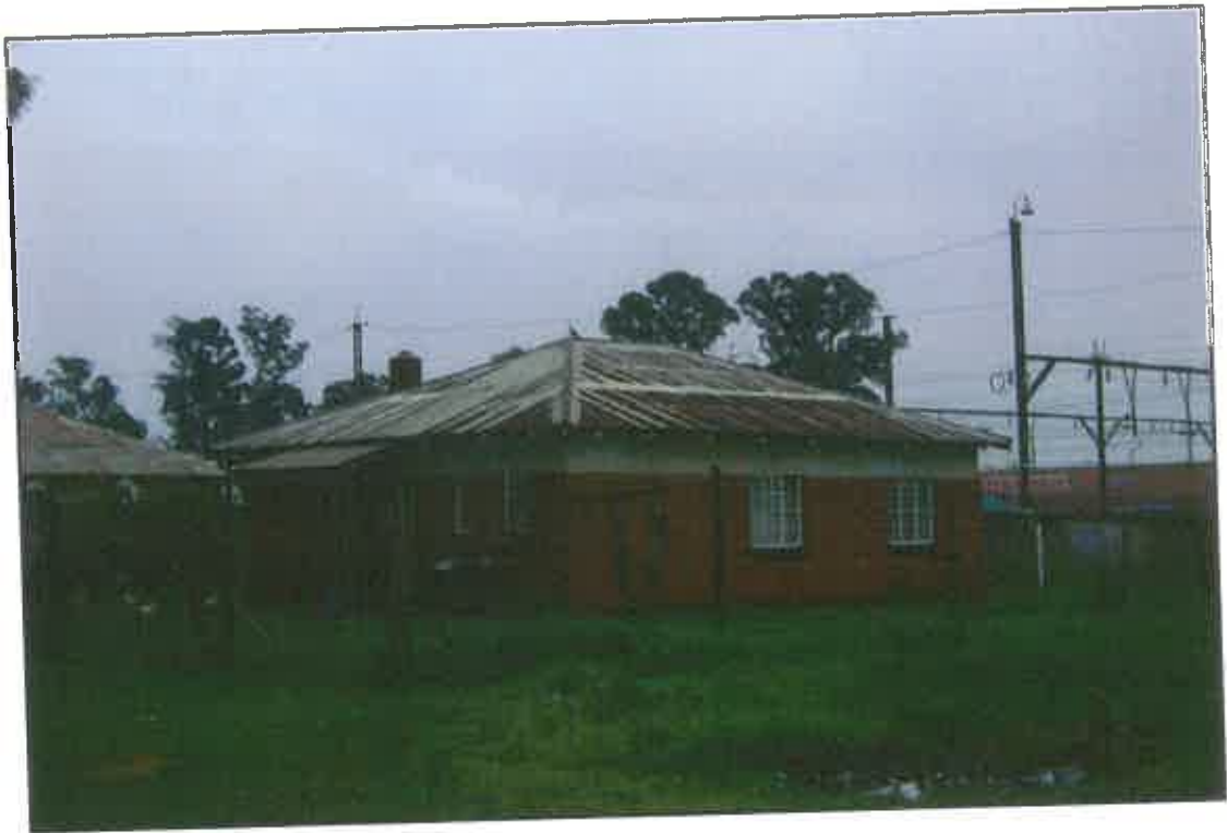
Figure 12. Typical station house at Delmas
