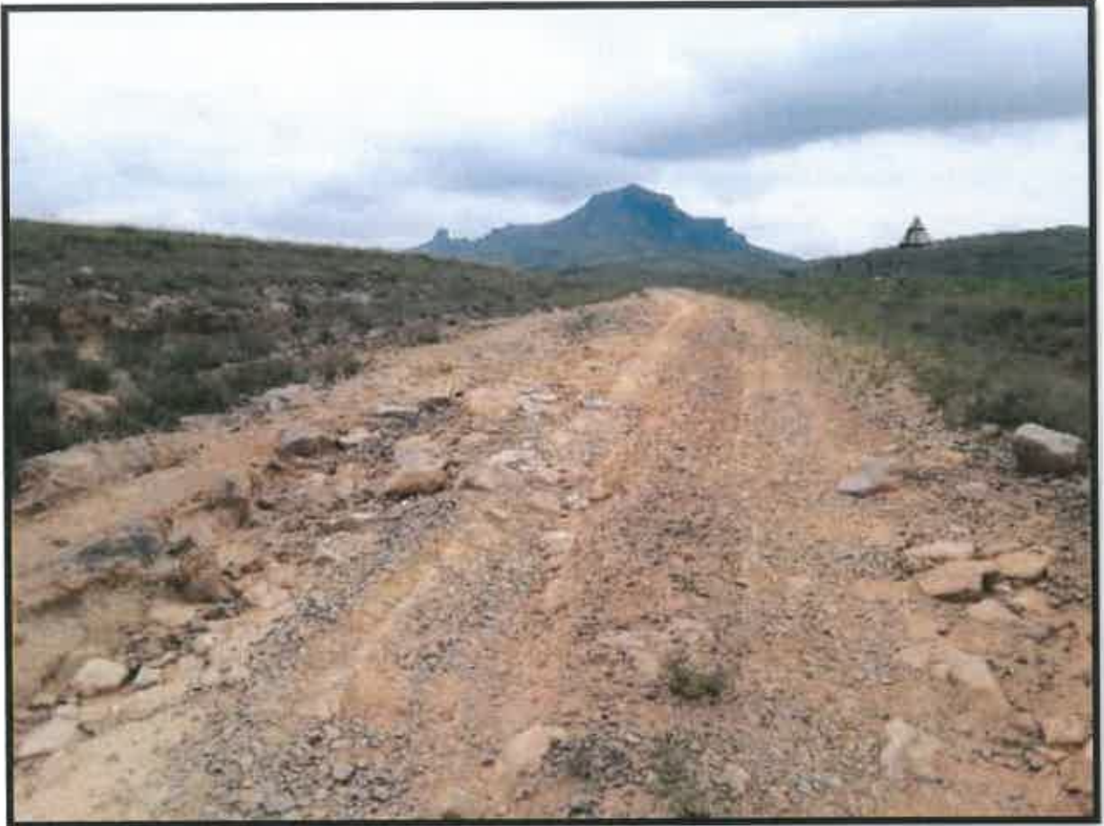
Figure 6: Road present on site.
