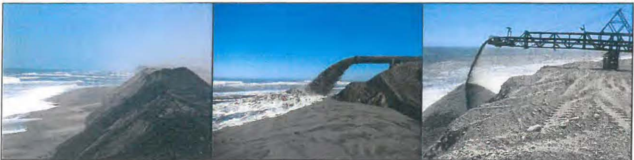
Figure 3.1: Beach accretion methods (left to right) - seawalls, dredger discharge, conveyor
