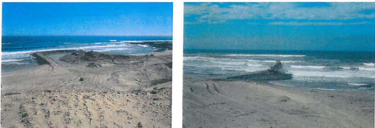
Figure 3.4: Rock berms used to reclaim mining area on the beach near Alexander Bay
