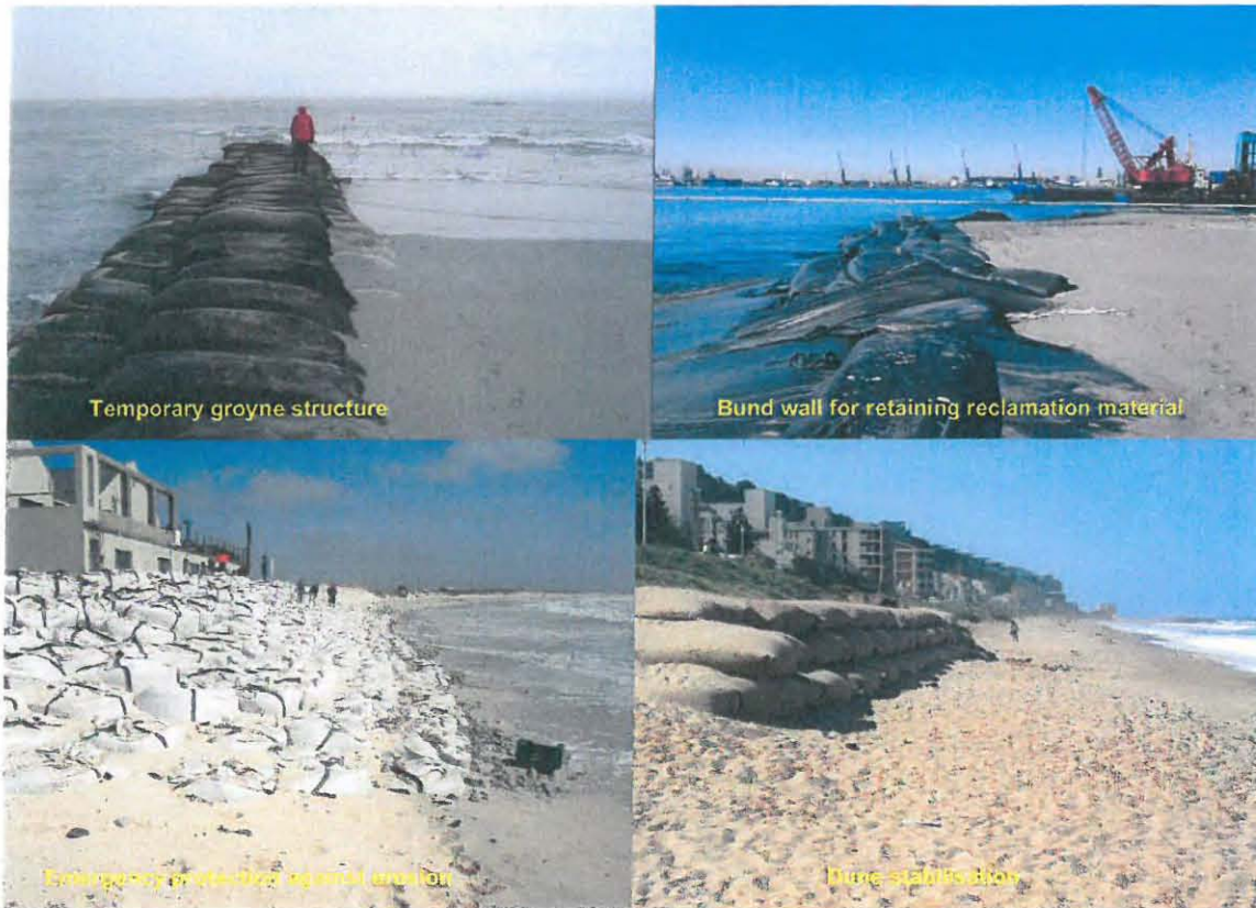
Figure 3.5: Applications of sandbags for coastal protection and reclamation works
