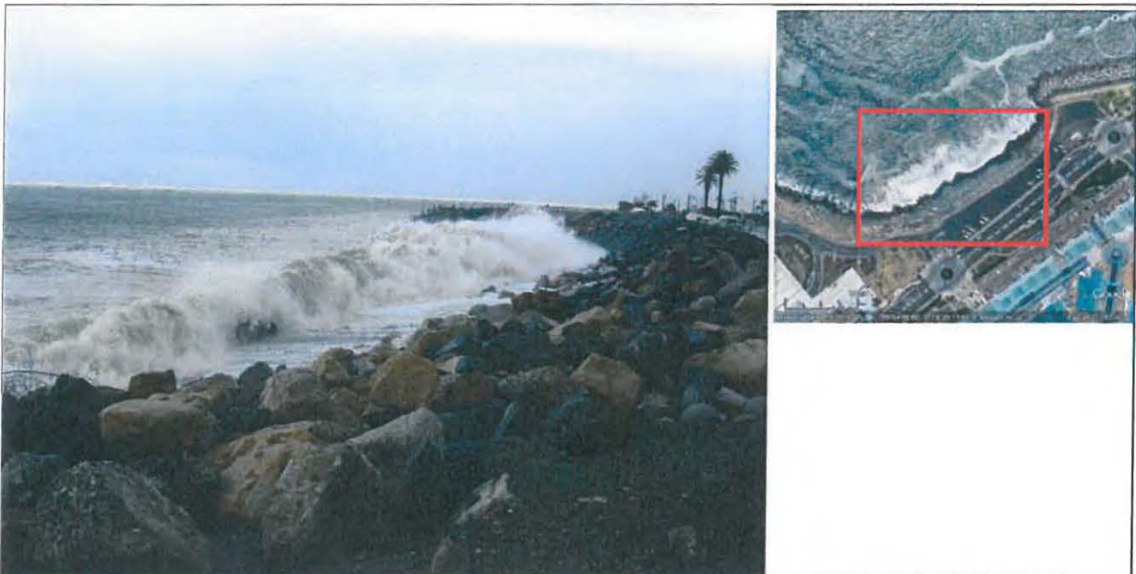
Figure 5.4: Example of a dynamically stable rock beach constructed for coastal protection at the V&A Waterfront, Cape Town
