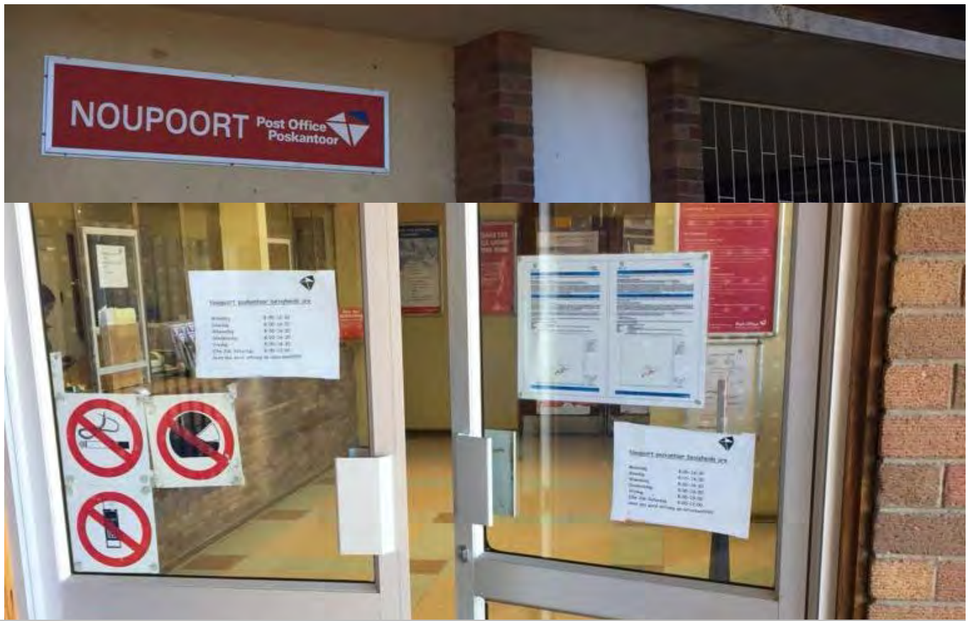
Noupoort Post Office
