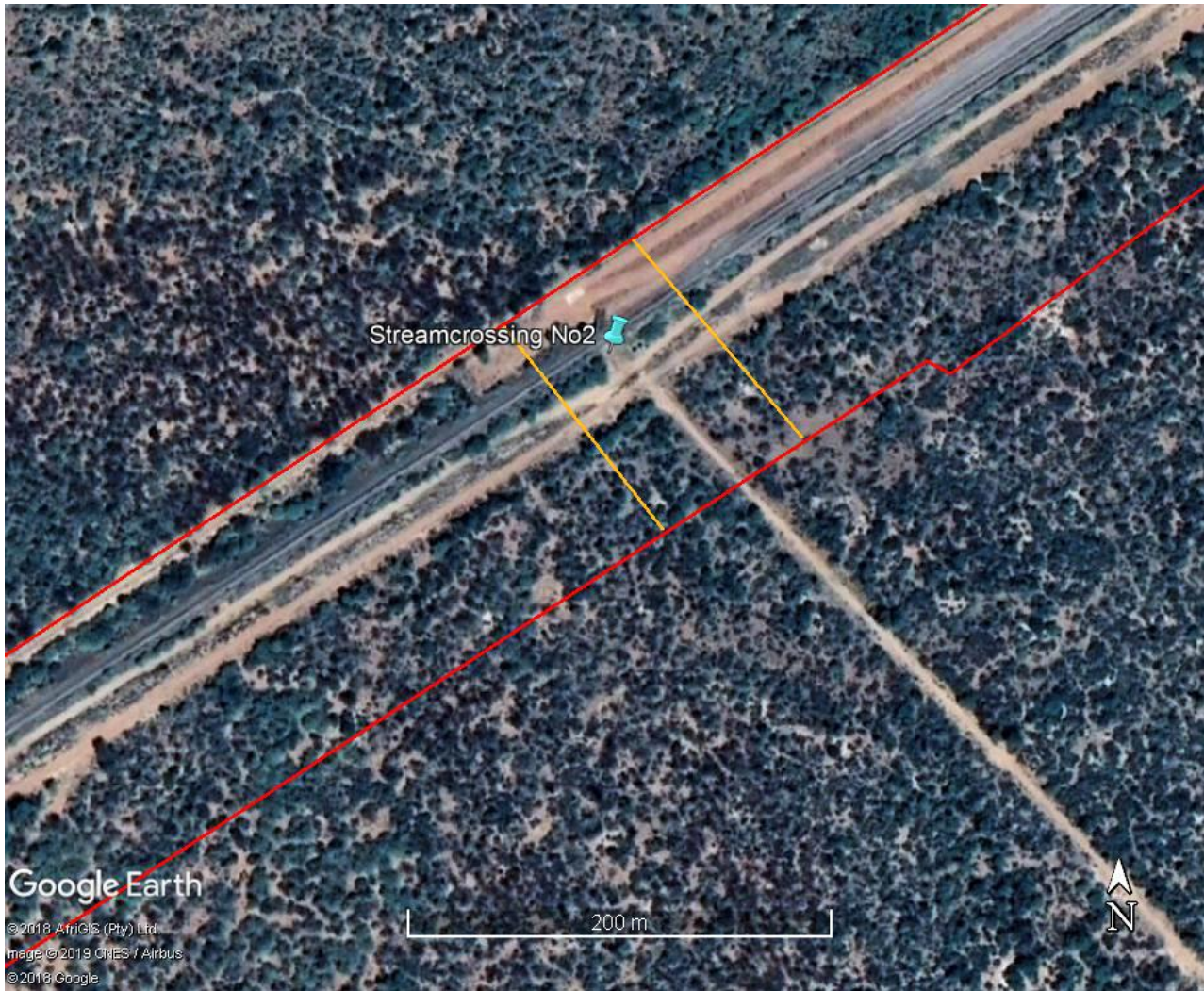
Figure 6 Indication of Streamcrossing No2 at the eastern parts of the proposed Railway Yard site.
