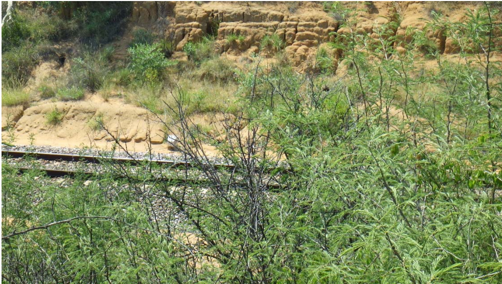
Figure 21: The railway line in the cutting will lower the visible disturbance at this point (KOP10).
