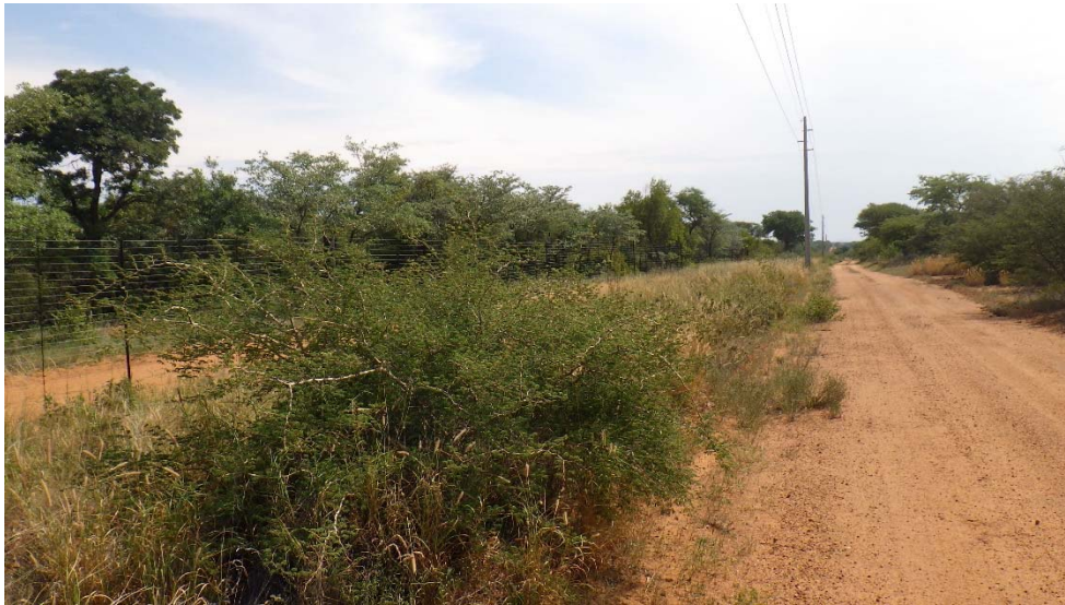
Figure 8: View of the section where the railway line is lowered – dense vegetation to the right screen the area.
