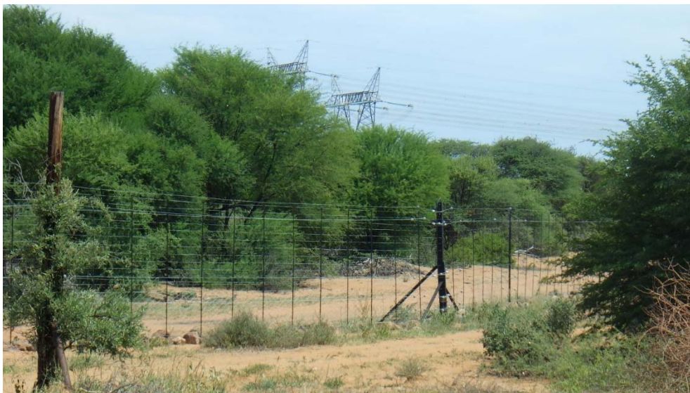
Figure 33: View from the railway access road towards the power lines near the boundary fence.
