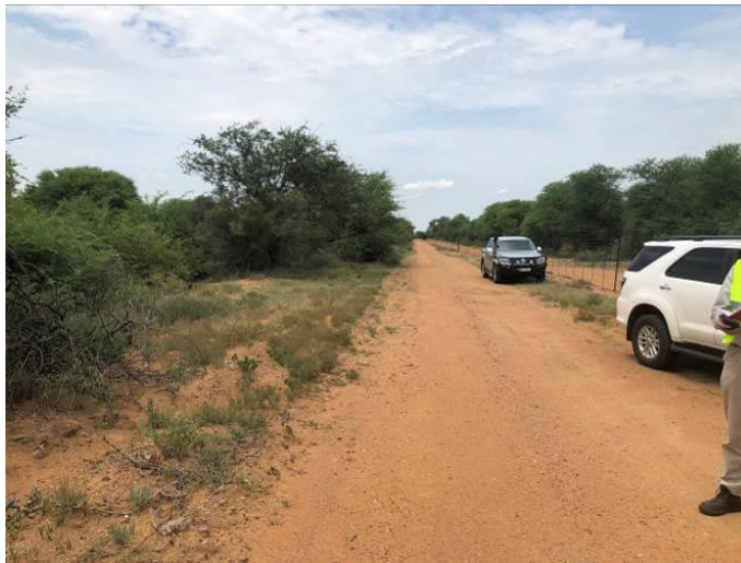
Typical section along the railway line (near the end of the yard)
