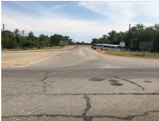
D26491 towards the Steenbokpan/Railway Yard
