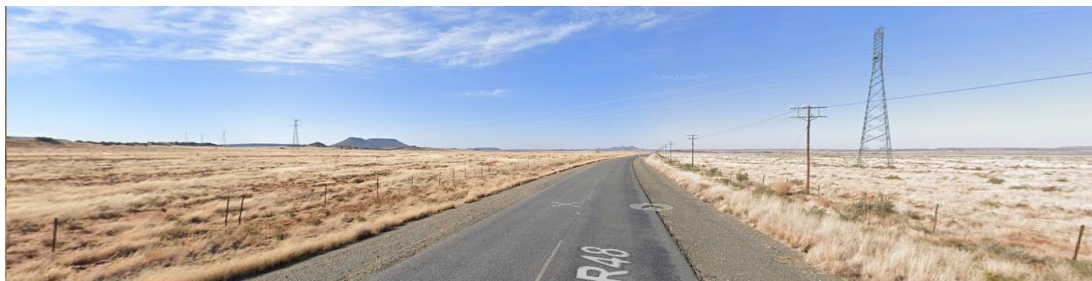
Figure 7: Powerline infrastructure within the study area (Photo: Google Earth)
