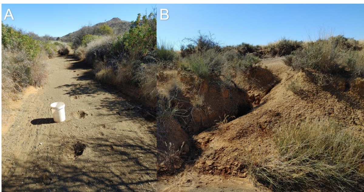
Figure 5-8 Photographs of features within the general PAOI: A) Dry river B) Drainage feature
