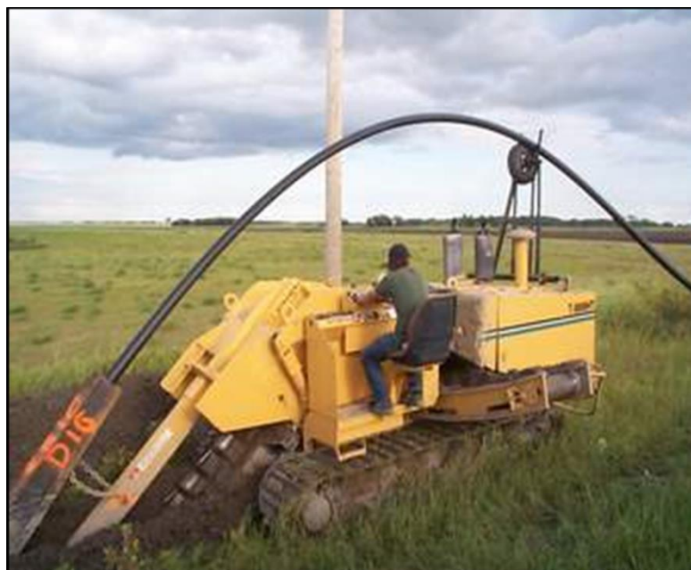
Figure 2: Typical excavator utilised for excavation of a trench.
