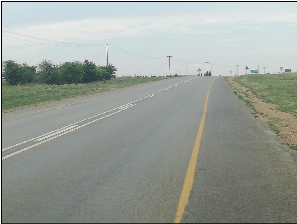
Figure 3: Road Access Along R30
