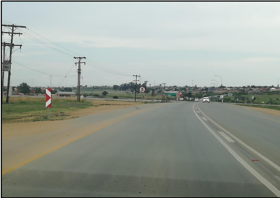
Figure 2: Overhead Power Lines at N14 - R30 Intersection
