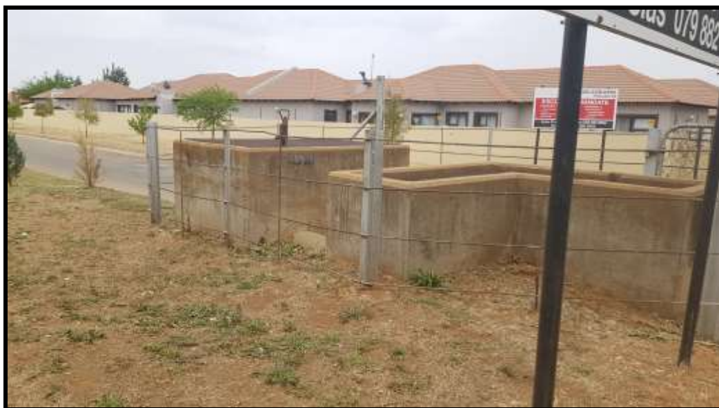
Photograph1: Sluice Gate to be removed
