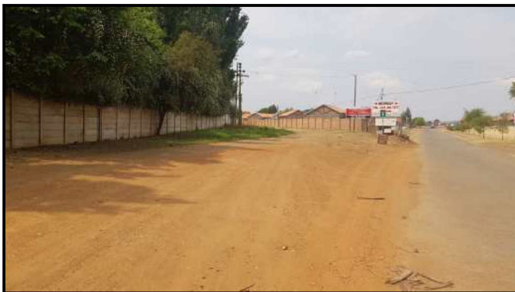
Photograph 2: Access road to be surfaced
