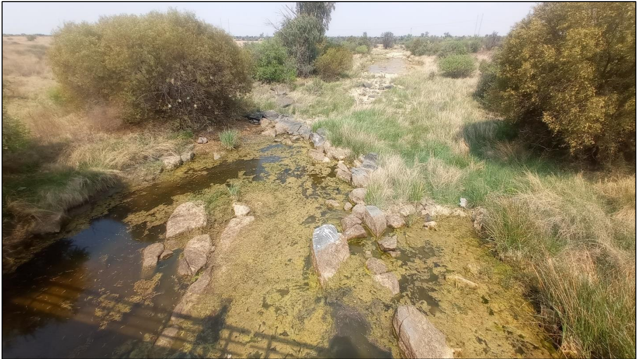
Figure 8-26: Channelled valley bottom of HGM 3 (October 2022)
