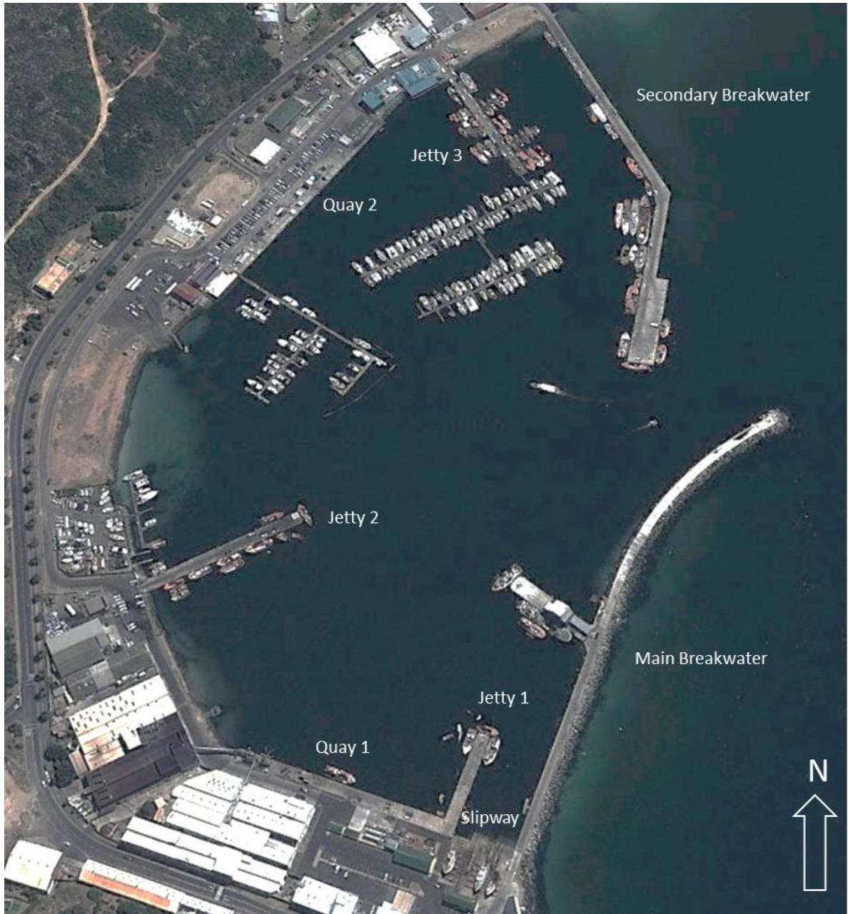
Figure 2-1: Hout Bay Marine Structures
