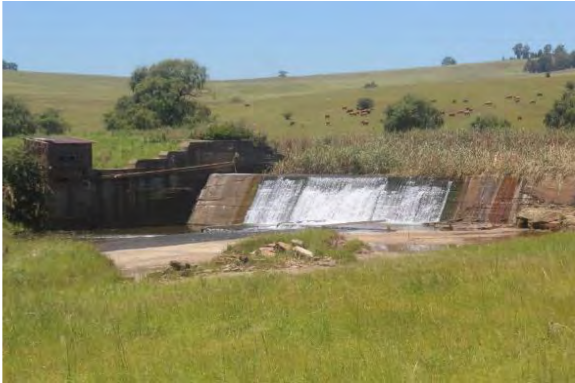
Figure 6.3: One of many drainage lines on the site.
