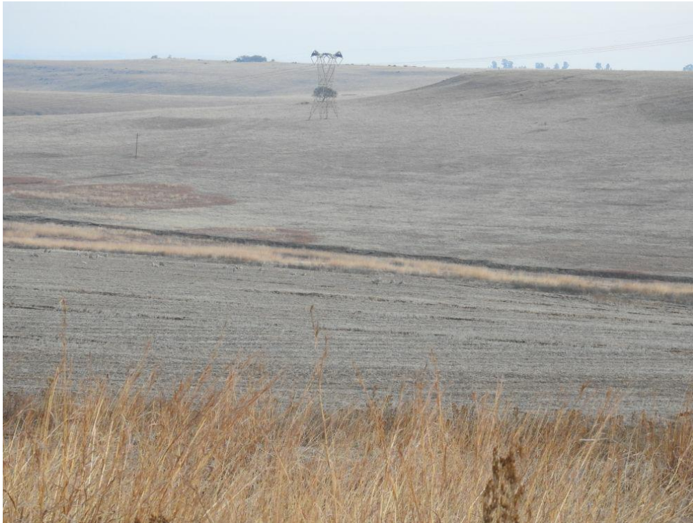
Figure 7: High voltage powerline at PAOI.
