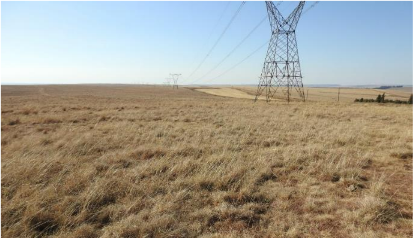
Figure 5: High voltage lines
