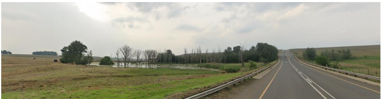
Figure 5-2: Riparian zone and vegetation adjacent to the N11
