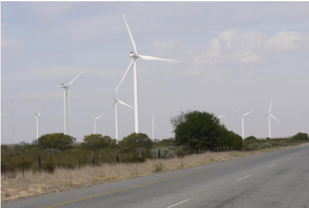
Plate 16, Hopefield Wind Farm from its immediate vicinity. The turbines dominate views.
