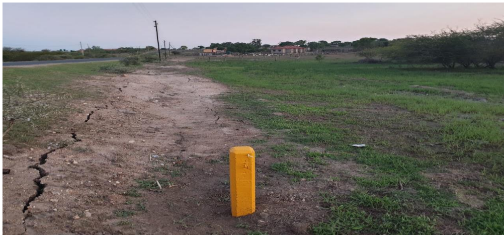
Figure 5: Picture of water pipeline installation activities that created cracks on the wetland
