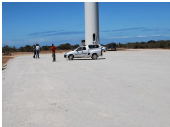
Figure 5-34: Example of typical wind turbine footprint (including lay down area and turbine footprint).
