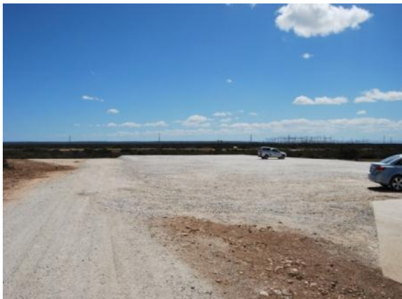
Figure 5-34: Example of typical wind turbine footprint lay down area (Coega IDZ).
