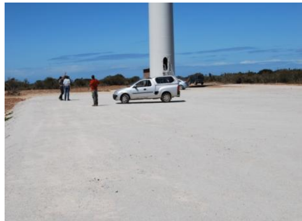
Figure 5-35: Example of typical wind turbine footprint (including lay down area and turbine footprint).
