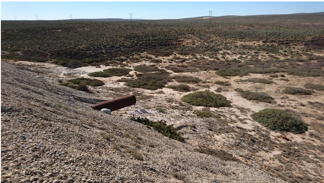
Photo g - 2: Photos of the main haul road situated 3 km upstream of the mouth within the restricted mining concession area of the WCR. This road prevents the river from reaching the floodplain. Photo A faces upstream and photo B shows how the intake pipe is elevated at least 1 m above the riverbed. Photos were taken on 23 June 2016.
