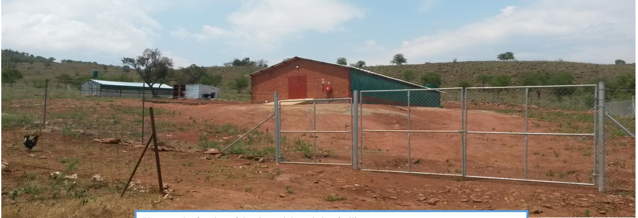
Photograph of portion of the site and the existing facility
