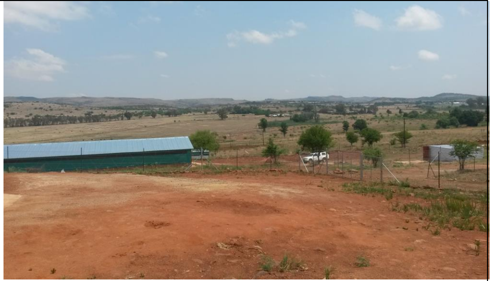
Figure 8 Photograph of site, showing bare/landscaped surface.
