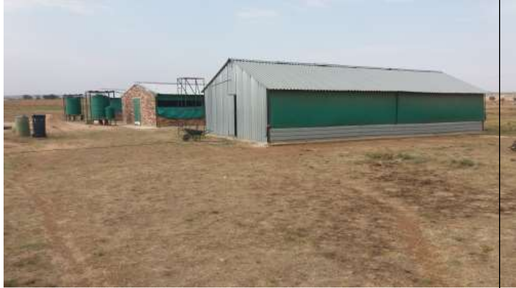
Figure 1 Some of the existing poultry houses
