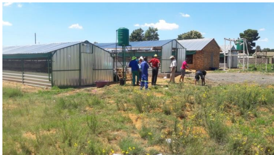
Figure 1 Some of the existing poultry houses
