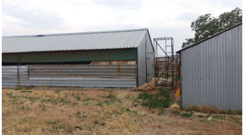
Figure 1 Some of the existing poultry houses
