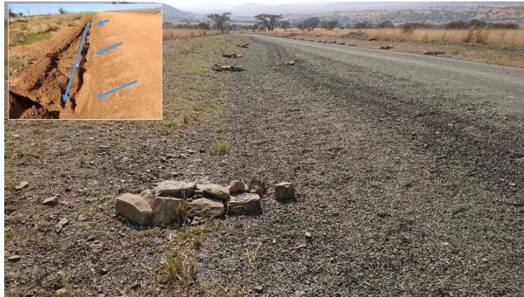
Figure 6-3 Example of road margin erosion prevention
