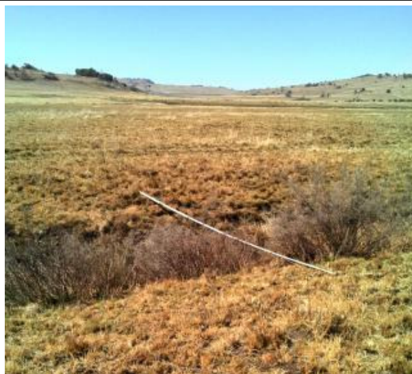
Figure 14: Gabion diversion wall, W42C-01-207-00, looking in a south-easterly direction
