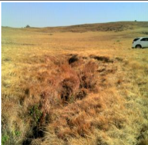
Figure 21: Road to be stabilised/protected by means of concrete strips and a gabion cut off wall (W42C-02-209-00) looking in south-westerly direction
