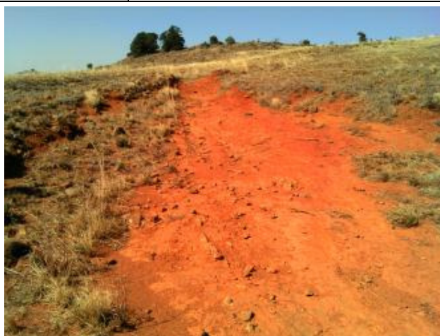
Figure 23: Erosion rehabilitation (intervention W42C-02-211-00) looking in a south-easterly direction
