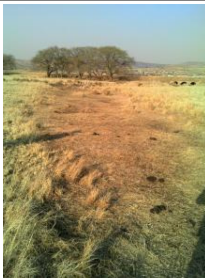
Figure 35: Channel to be excavated (V31A-01-201-01), looking in a north-easterly direction
