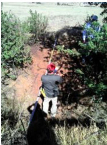
Figure 11: Reno mattress, WC42-01-205-00, looking in an easterly direction
