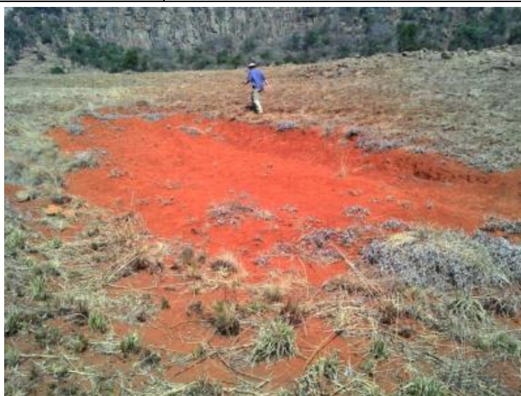
Figure 26: Hillside erosion rehabilitation (intervention W42C-02-215-00) looking in a north-westerly direction
