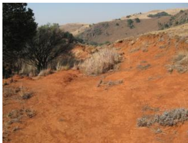
Figure 27: Gully to be rehabilitated (W42C-02-215-00) looking in a south-easterly direction
