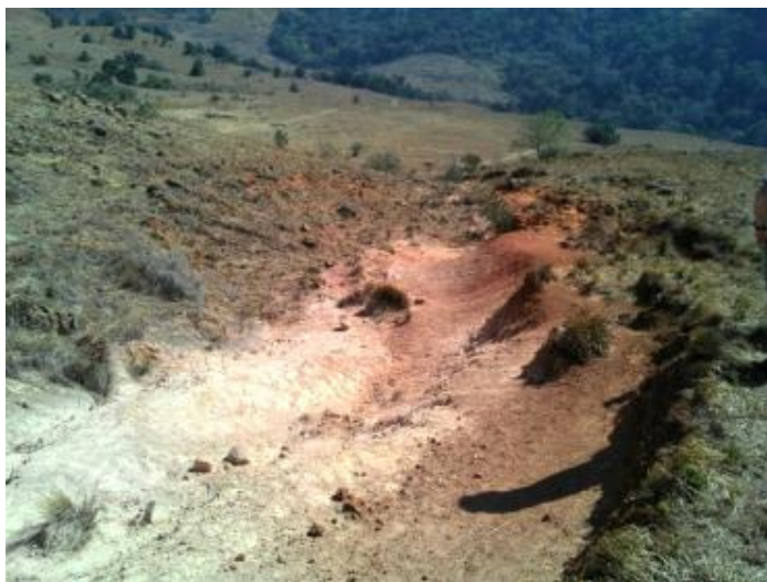
Figure 24: Erosion rehabilitation (intervention W42C-02-212-00) looking in a north-westerly direction
