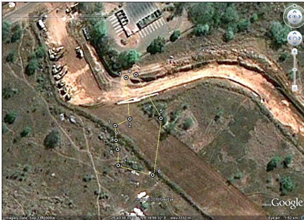
Figure 3. The original cemetery boundaries indicated in archival sources , on which the excavations were based, transposed on the Google Earth image of the site. The pipeline construction activities and the damage to the cemetery are clearly visible.
