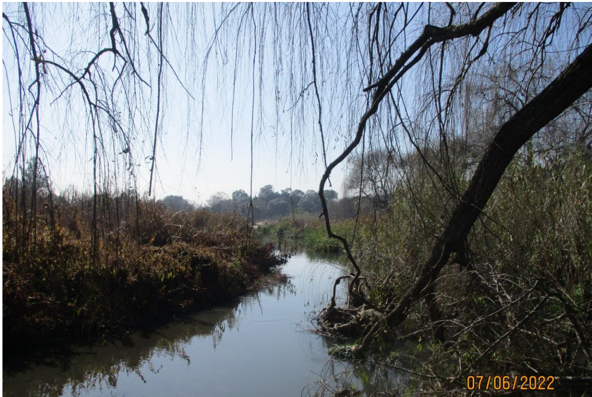
Figure 7-3: The current state of the Watercombe Dam
