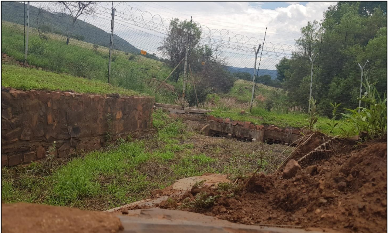
Figure 8: A non-perennial channel in vicinity to the Proposed Eskom Powerline Lomond-Safari.
