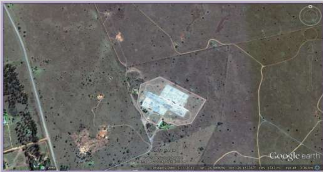
Figure 1: Watershed Substation (Google; 2013)
