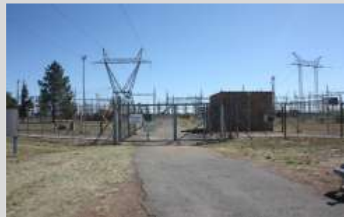
Figure 3: Existing access road on site (Aken: 2014)
