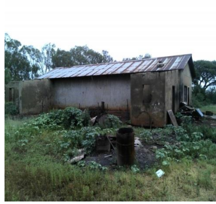
Dwelling viewed from the south.
