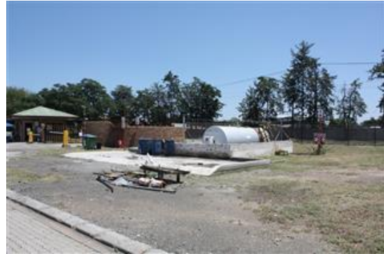
Above-ground diesel storage and refuelling area
