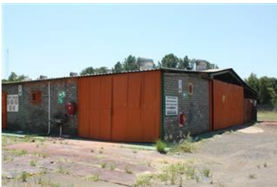
Hazardous substance storage areas (e.g. Paint store)
