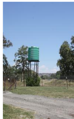
Potable water tank
