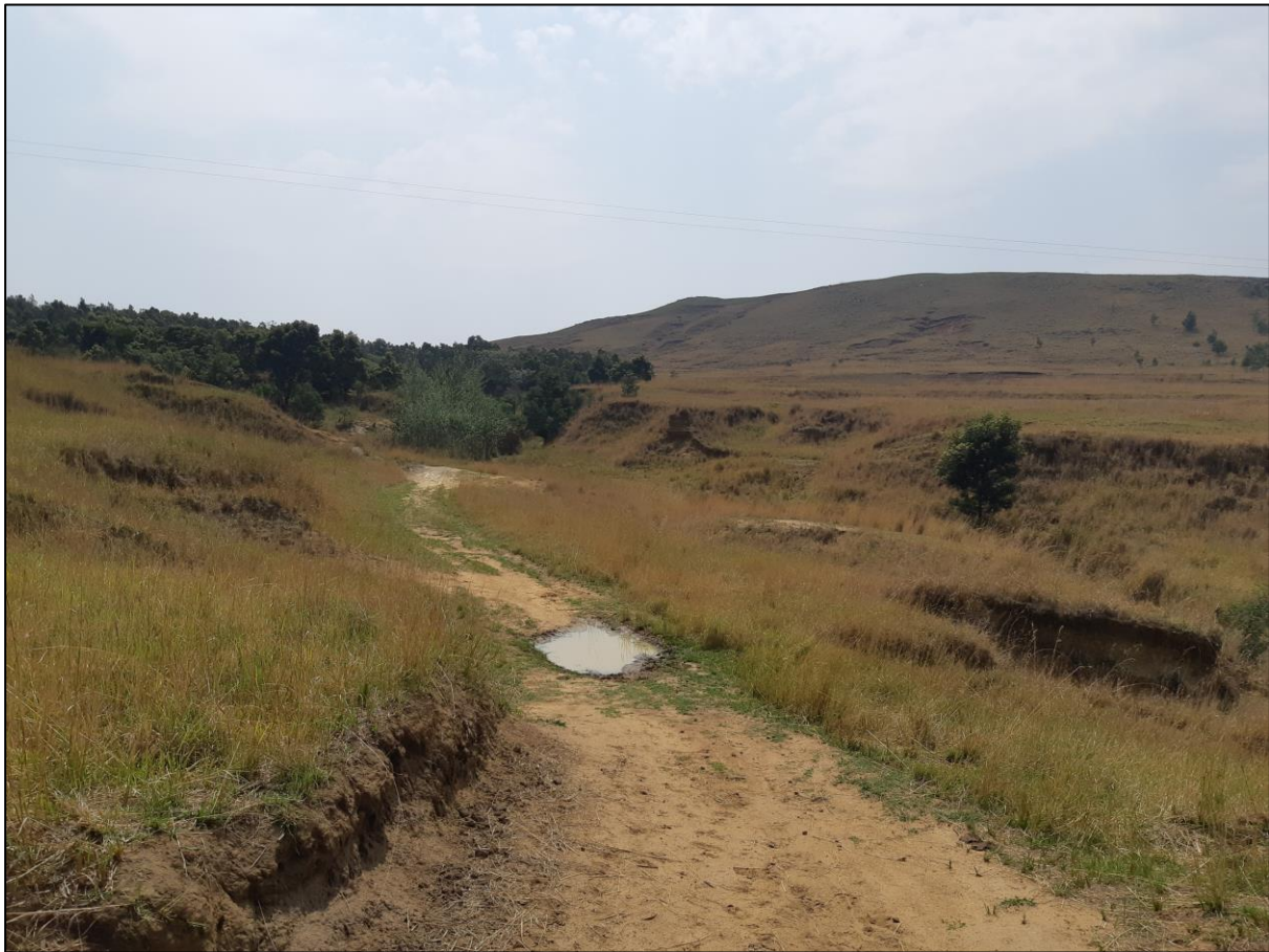
Figure 9: One of the crossings (Crossing 1) and the current road
