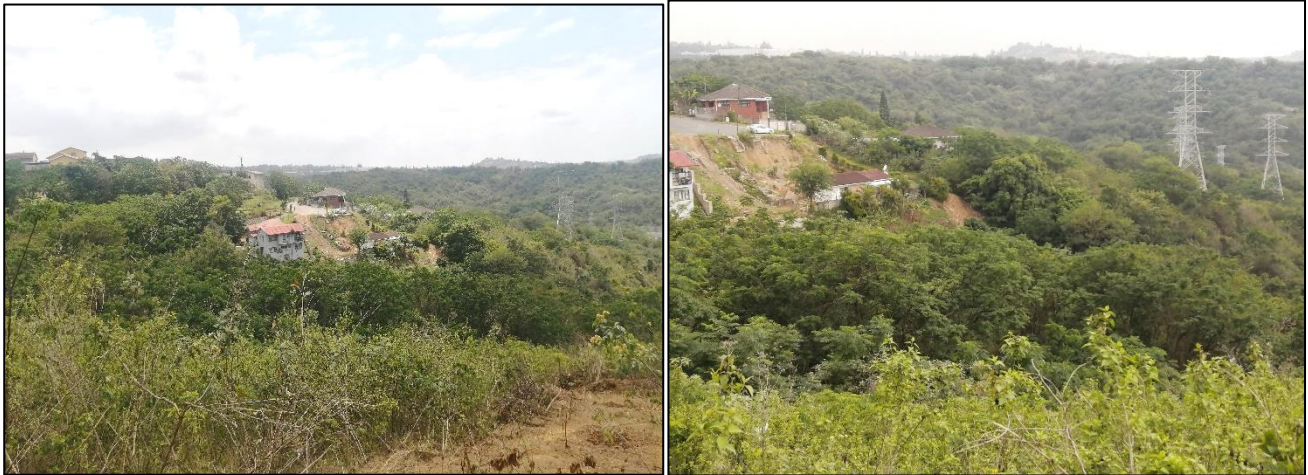
Figure 5: Drainage line across the development footprint.
