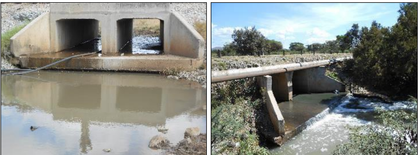
Figure 71: Culvert Bridge indicating elevation drops at biomonitoring sites.
