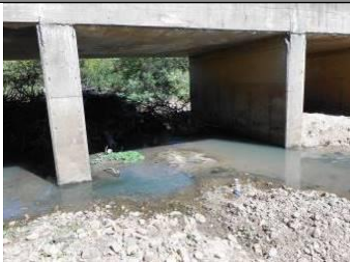
Figure 51: Upstream view of the SASS 31 site indicating the low flow and discoloured water at the time of the assessment likely due to presence of untreated sewage effluent.
