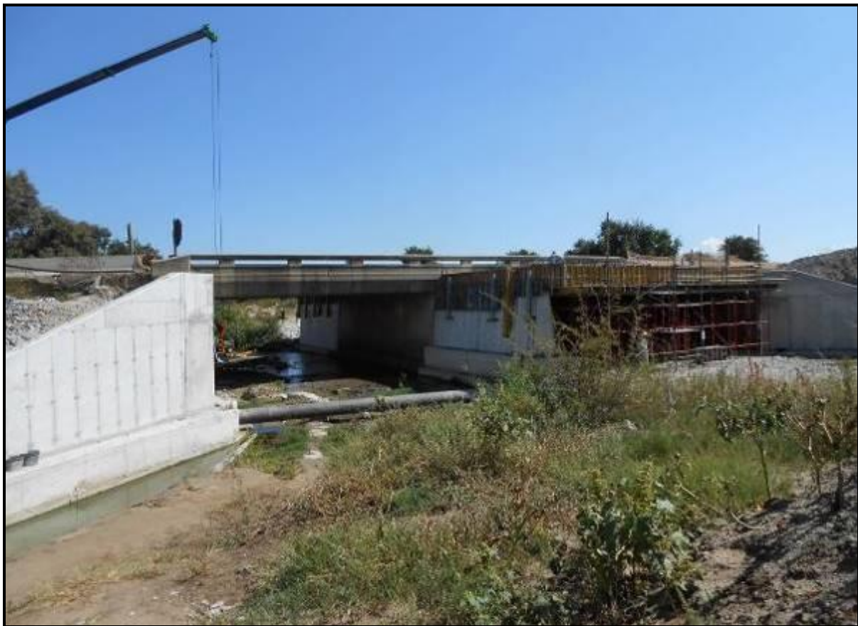
Figure 14: Representative photograph of the construction activities within the Dorpspruit
