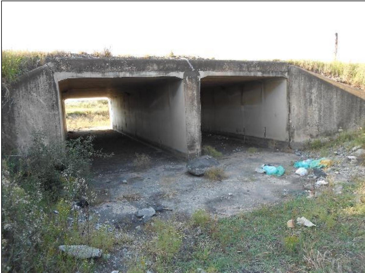
Figure 67: Culvert Bridge indicating the artificial habitat within the structure.
