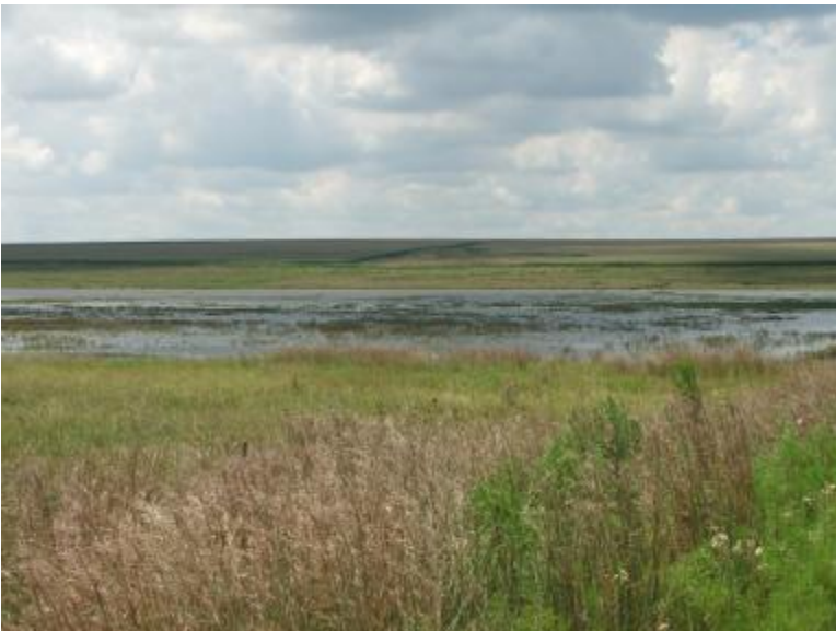
A view of a dam used for agricultural purposes
