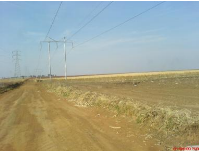
A road and power line transecting the pan on the northern boundary.
