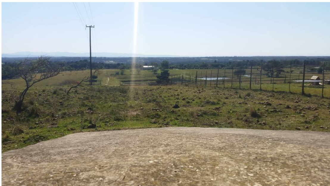
Figure 16: The series of dams in the background as seen from the gate at Spruce Rd.
