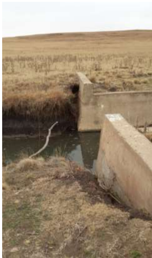
Figure 29: Intervention site C81H-11-204-01.
