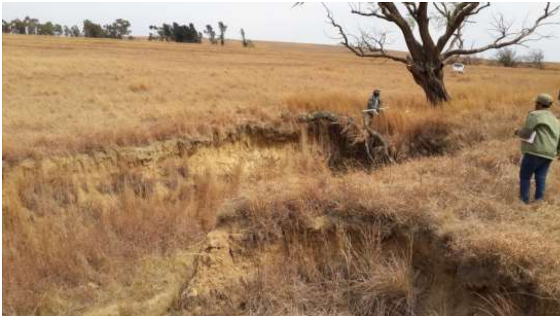
Figure 10: Intervention site C81D-01-204-00 looking upstream.
