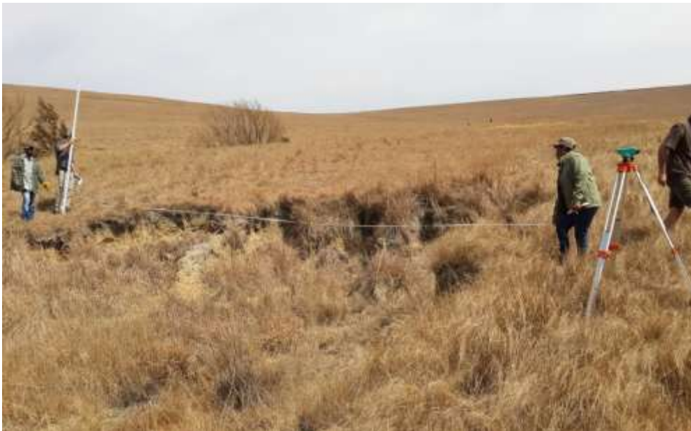
Figure 9: Earthen diversion berm, C81D-01-203-00 looking upstream.
