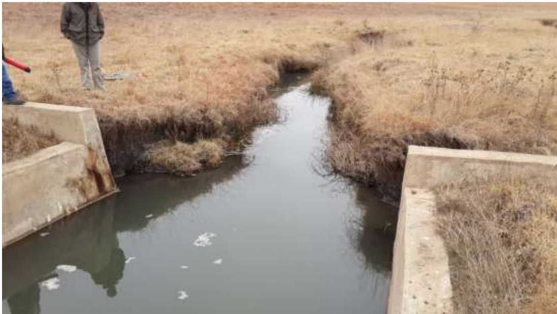
Figure 27: Intervention site C81H-11-202-01
