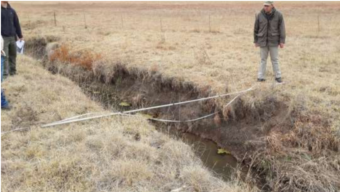
Figure 30: Intervention site C81H-11-201-00 looking upstream from the right bank.
