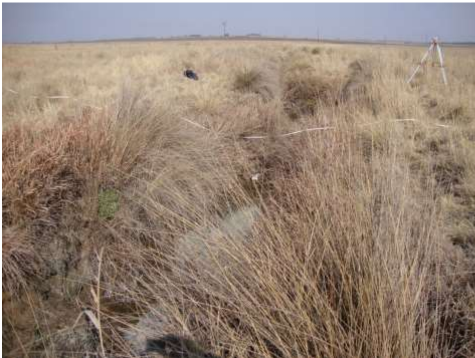
Figure 13: Stone masonry drop-inlet weir, B20G-01-220-00
