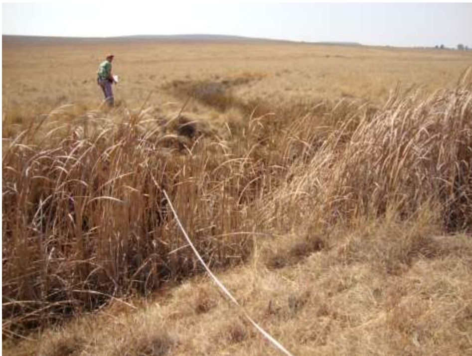
Figure 10: Stone masonry drop-inlet weir B20G-01-217-00
