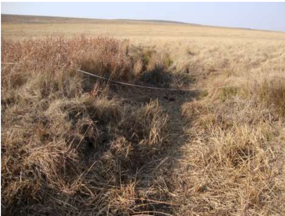
Figure 18: Earth structure (earthen berm) and re-vegetate, B20G-01-225-00
