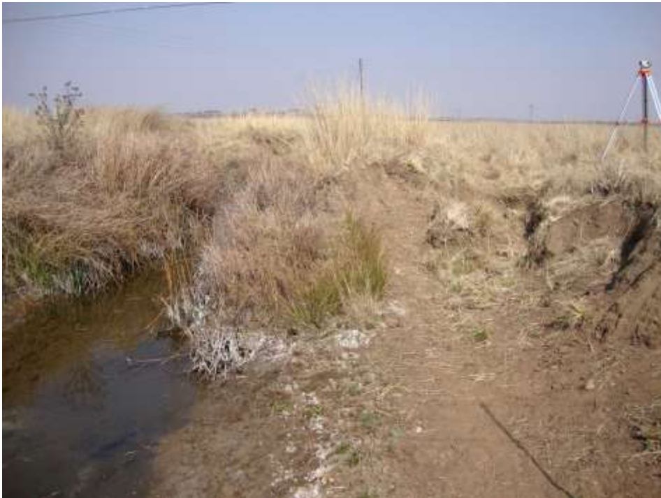
Figure 12: Stone masonry drop-inlet weir, B20G-01-219-00
