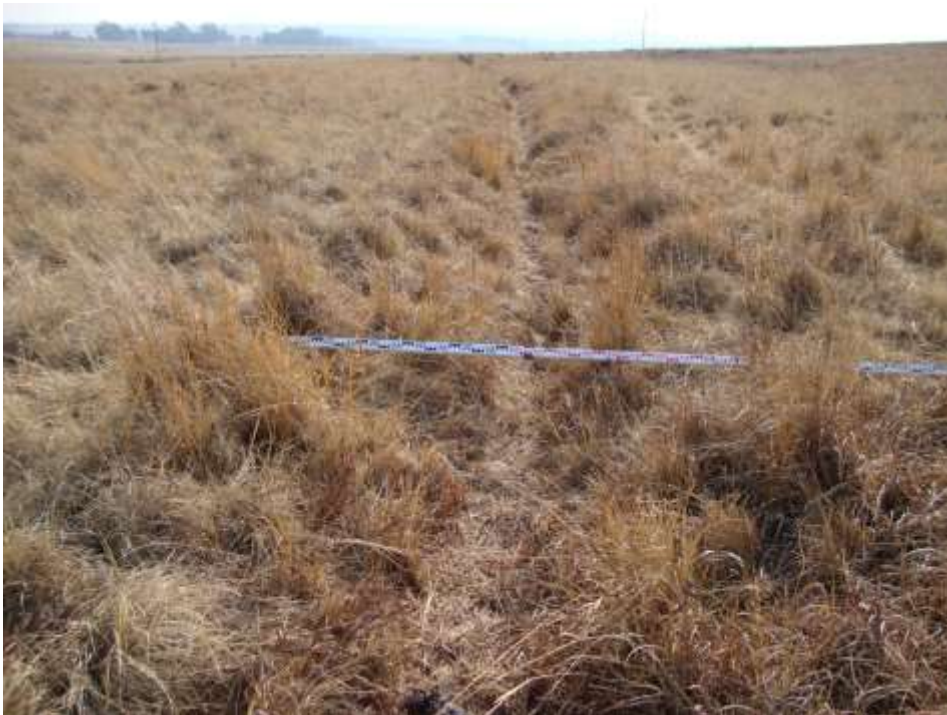
Figure 15: Earth works (cut & fill) and re-vegetate B20G-01-222-00
