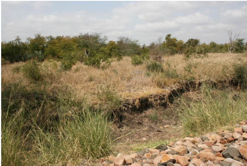
Figure 13: Site of intervention B90E-01-203-00
