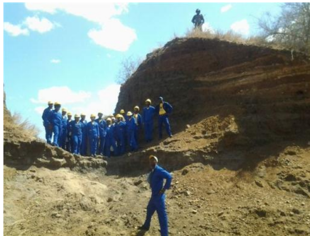
Working for Land team widening the existing breached area
