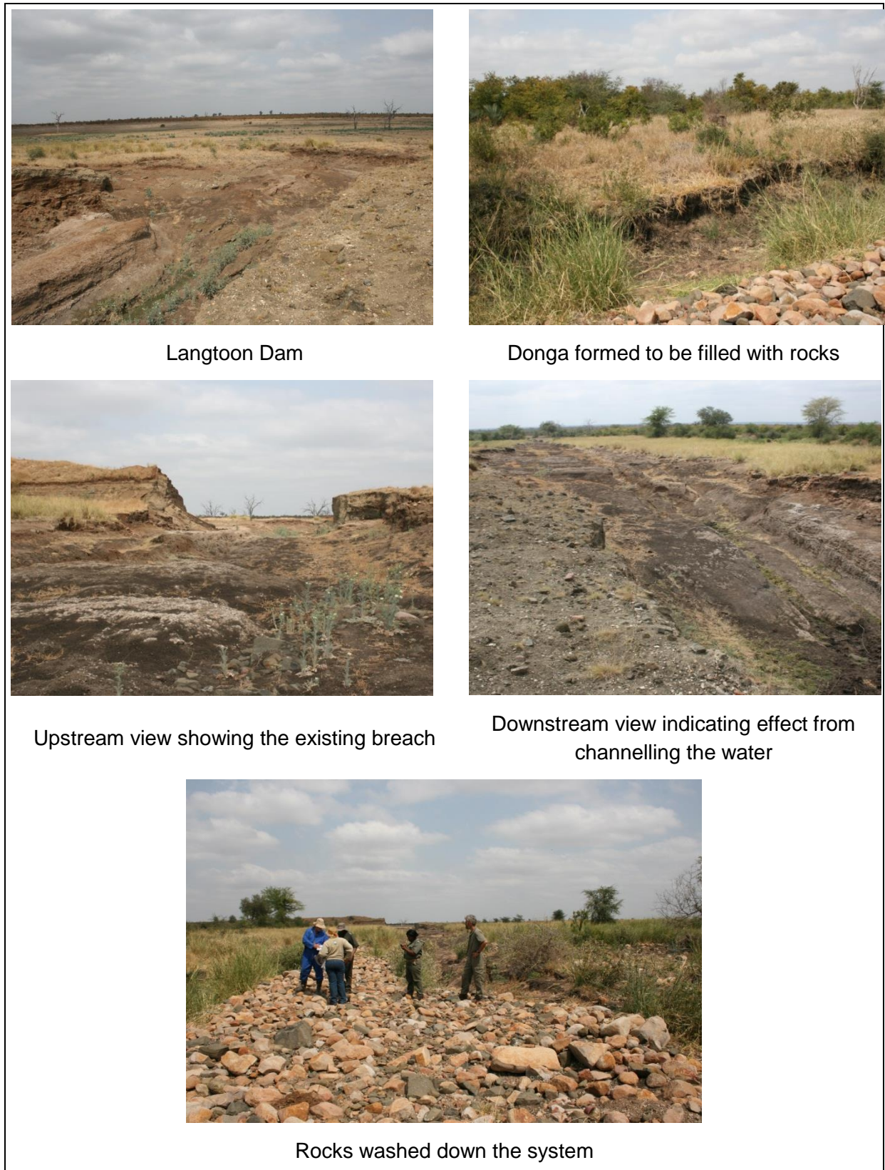
Figure 9: Site Photos of the Langtoon Dam Wetland
