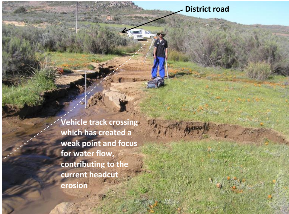
Figure 19: Headcut erosion in a road crossing the Langvlei wetland (Courtesy: Donovan Kotze)
